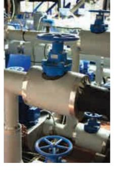
The complex system of pumps, pipes and valves that makes it possible to cool single zones of the extrusion line
